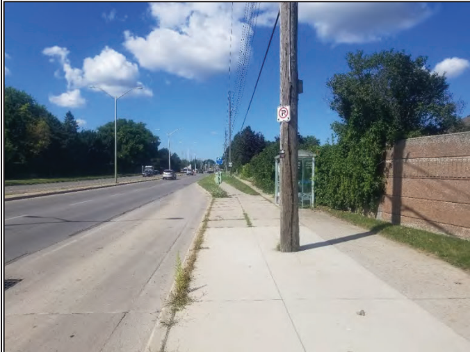
Photo 11: Typical ROW disturbance with residential sound wall along Richmond St, facing north
