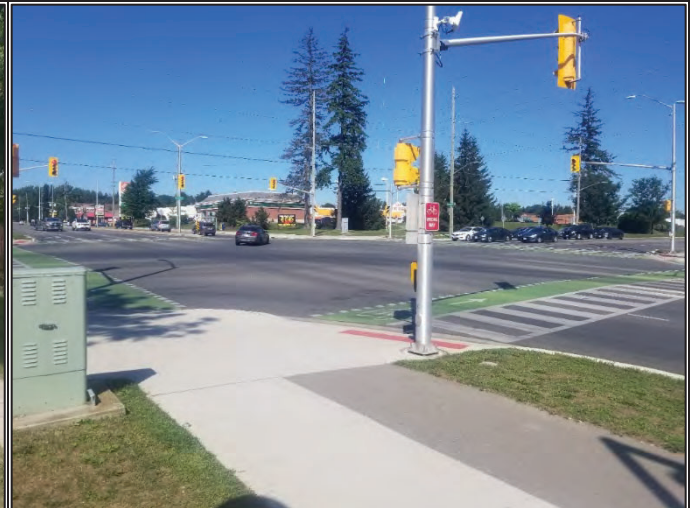
Photo 10: Typical intersection infrastructure disturbance, facing northwest
