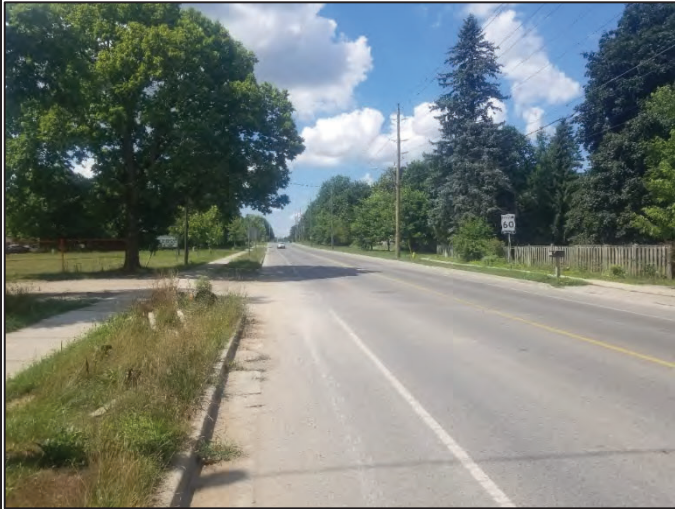
Photo 17: Existing conditions along Windermere Rd, facing west
