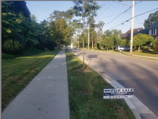
Photo 23: Existing conditions along Huron St ROW adjacent to residential structures, facing west
