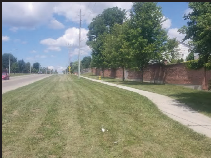
Photo 9: Existing conditions of Adelaide St ROW utilities and disturbance, facing northeast
